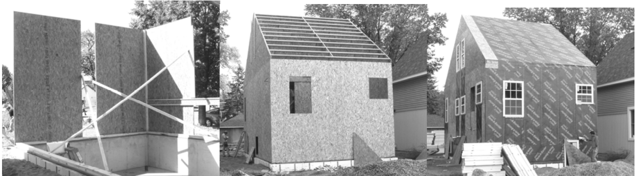
Fig. 4 house Two: corner panels and one joist ; all panel, windows and rafters in place membrane and windows await insulation
