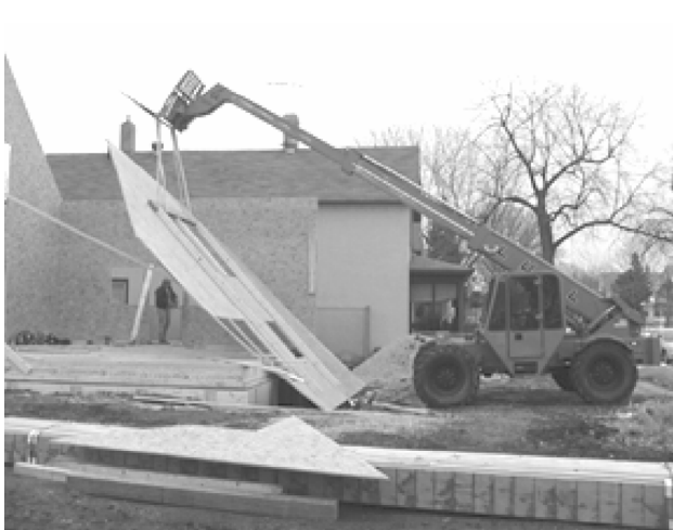
Fig. 2 Pilot House (House One) Lifting the gable end wall
