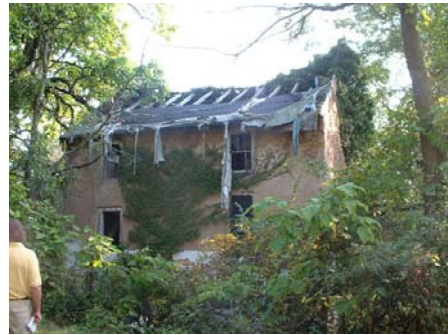
Fig. 6 Spring House Project
