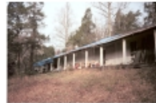
Figure 7. "Memphis Row", Yellow Sulphur Springs. Photo by author.
