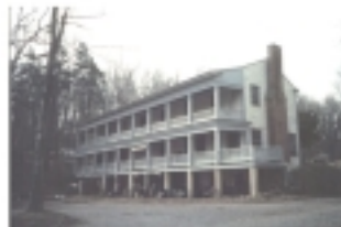
Figure 6. Yellow Sulphur Springs Hotel, Photo by Author.
