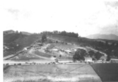
Fig. 4 An early photograph of the Tazewell Fairgrounds. Note the tunnel under the first turn. (Library of Virginia)
