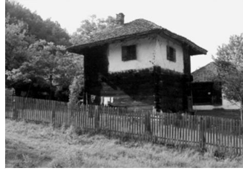
Elevation to land and valley below
