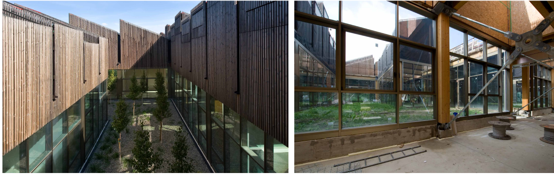
Figure 3: Interior courtyard (left); view to courtyard under construction (right). Source: (Moreno Maggi Photographer, MCA, 2017)
