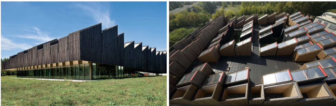
Figure 1: South and east facades (left); roof under construction (right). Source: (Moreno Maggi Photographer, MCA, 2017)
