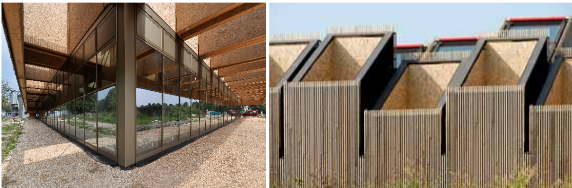
Figure 6: View of layered façade (left); roof under construction (right). Source: (Moreno Maggi Photographer, MCA, 2017)
