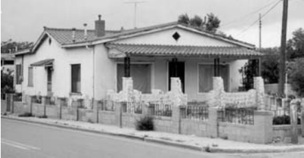
Figure 12 Residence at 707 Agua Fria Street
