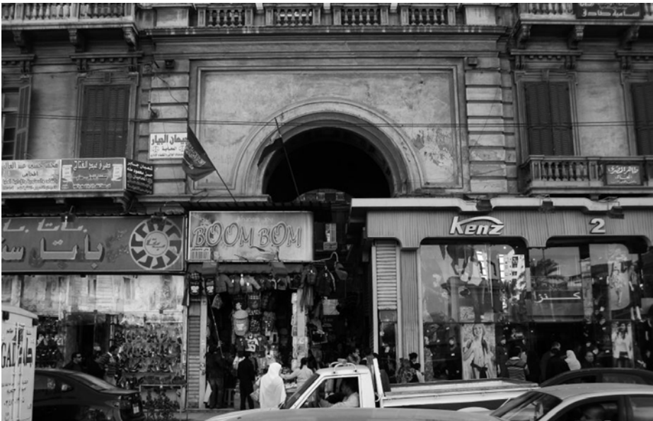
Figure 1: Main entrance to Okelle Mensesce from Mansheiya Plaza showing adjacent shops encroaching on entrance and non-harmonious shop facades (2010).
