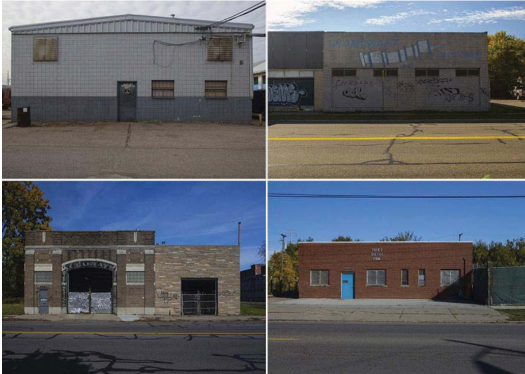
Figure 1: Street views of operational Detroit fabrication shops, Fall 2012. Source: ( Re:Tool-Kit for Detroit , 2012)
