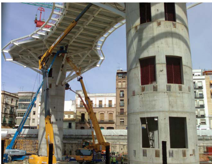
Figure 2. The Metropol Parasol under construction Photo by Torchondo.
