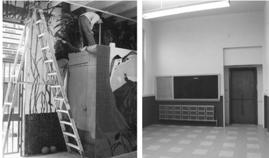
Fig. 2. Art-making in the community spaces. a) Mural in daycare center, b) Church kitchen renovation.
