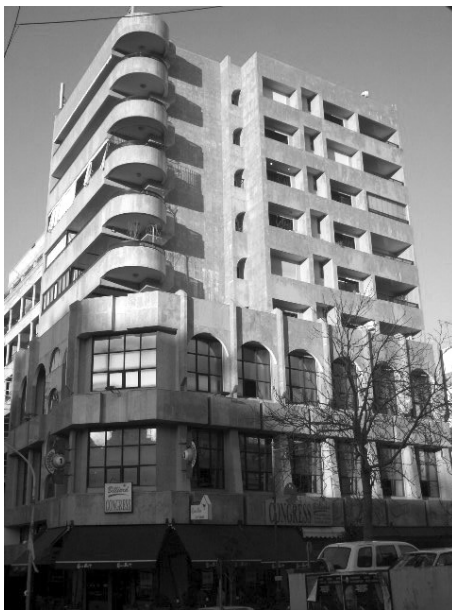
Figure 3. Apartment Buildings, Beirut
