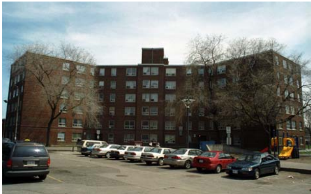
Figure 3: Regent Park North, 6-story "dogbone" building, courtesy Toronto Community Housing Corporation
