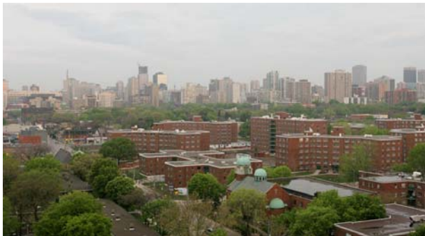
Figure 5: Regent Park Phase I redevelopment parcel, pre demolition, courtesy Toronto Community Housing Corporation (TCHC)
