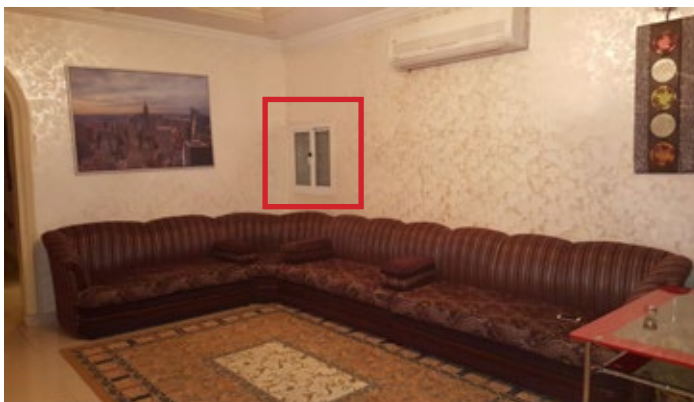
Figure 4a. Light well windows in the living space. (third floor).
