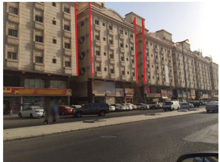
Figure 1. Small gap between buildings in Jeddah
