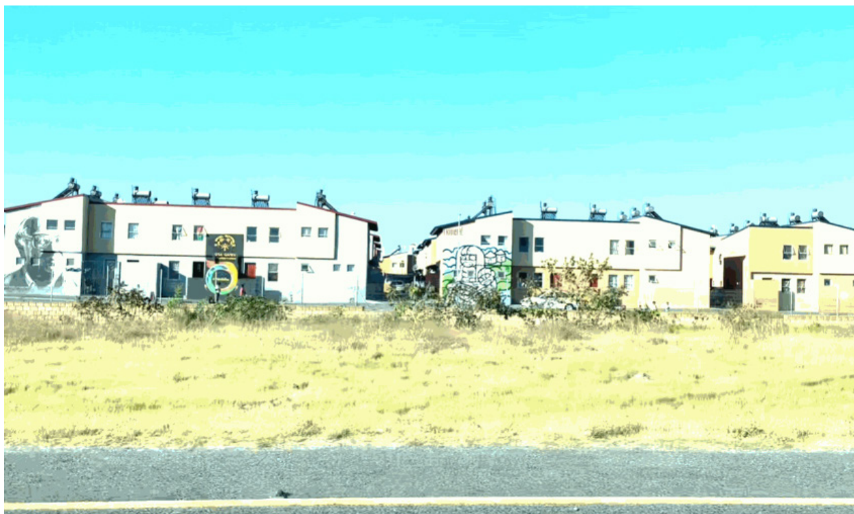
Figure 3: Solar Water Heaters have been installed on the roofs of Cape Town’s N2 Gateway Housing project. Opportunities in the built environment to better equate local need with decentralized water and energy systems requires cross-sector collaboration, the provision of subsidies, training for local installers and distributors, and community participation. (Author’s Image).
