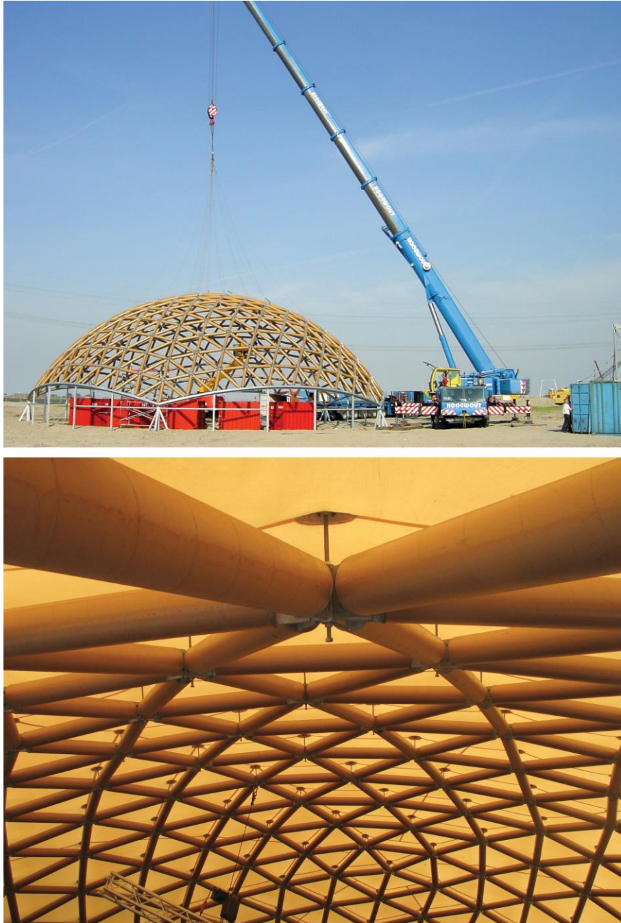
Figure 13. Paperdome's assembly process and interior view detail showing steel joints. Source: Octatube Engineers
